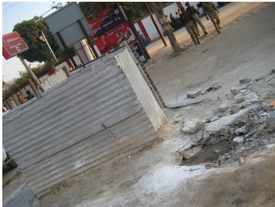
Figure 15: Zero Discharge Toilets
